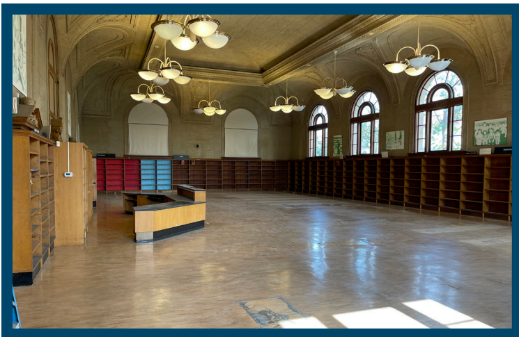
Ready for construction at the San Francisco Public Library Mission Branch
