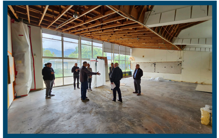
Under construction at Ventura County's Meiners Oaks Branch Library
